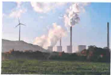
A coal-burning power plant steams in Gelsenkirchen, Germany while the 23rd UN Conference of the Parties (COP) climate talks end in Bonn, Germany, Friday, Nov. 17, 2017. (AP Photo/Martin Meissner)
